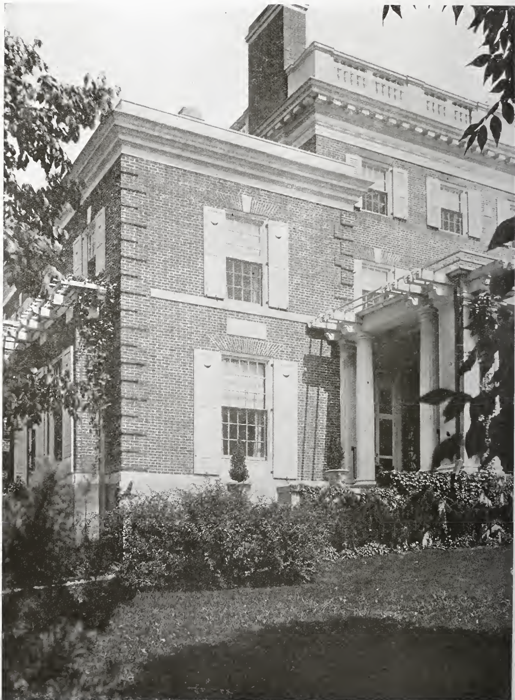
DETAIL—RESIDENCE OF GEORGE L. NICHOLS, ESQ. Katonah, N. Y.
